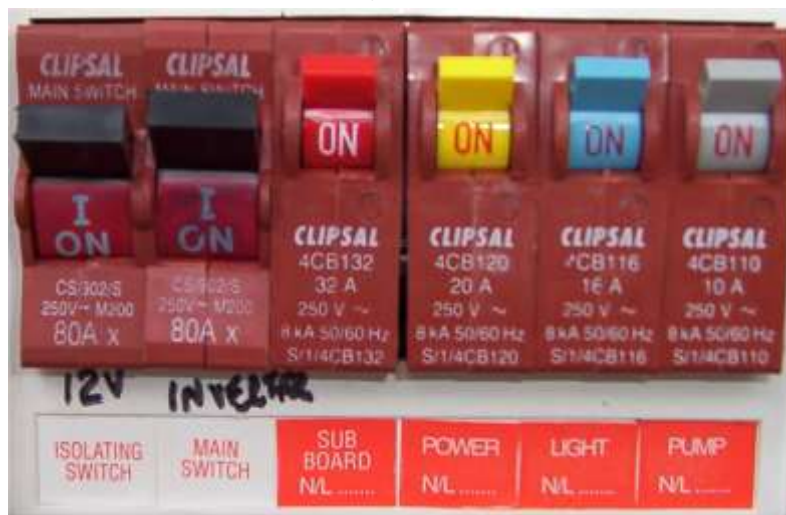
Figure 35 - D.C. Power On, Inverter On
